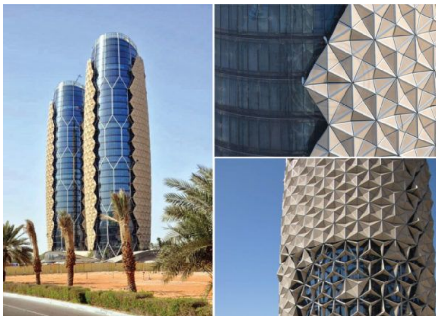
Figure 3 – Abu Dhabi Investment Council ‘Al Bahar’ building in Abu Dhabi, UAE
