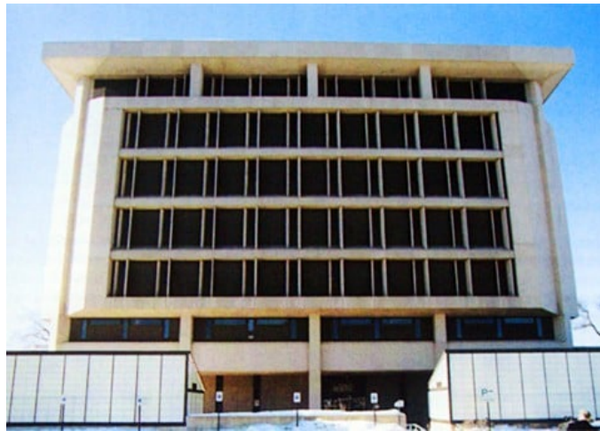
Figure 1 – The first energy efficient building in Manchester (USA)
