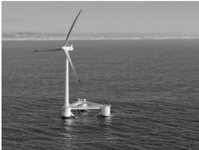
Figure 5. Floating WPP in Japan 23 km from Fukushima
