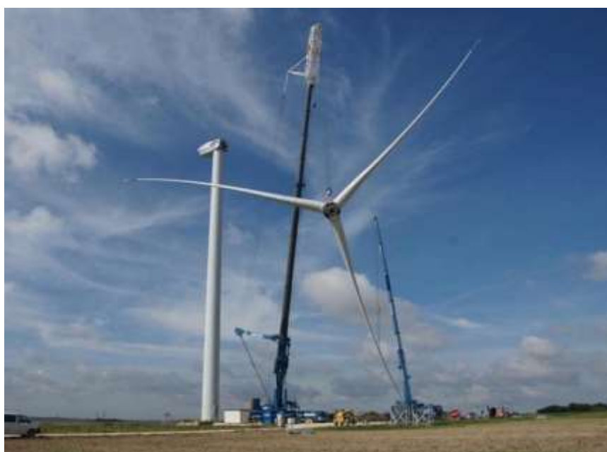
Figure 3. The process of installing a wind generator
