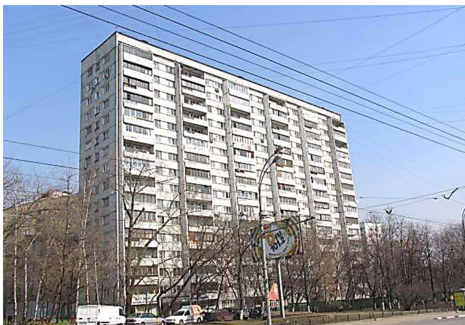
Figure 1. Sixteen-storey frame-panel house of the 1MG-601D series
